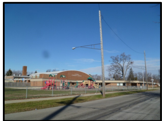
Figure 17: View from Washington Street
