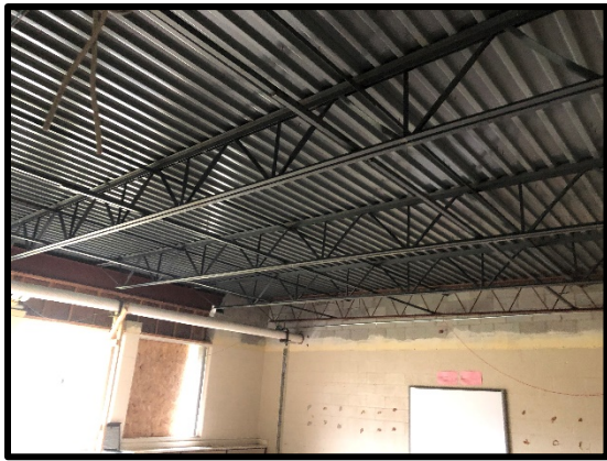
Figure 20: Roof Construction at addition
