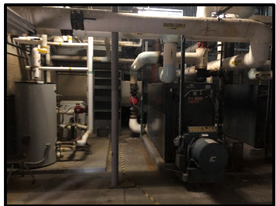
Figure 23: Main Mechanical Room
